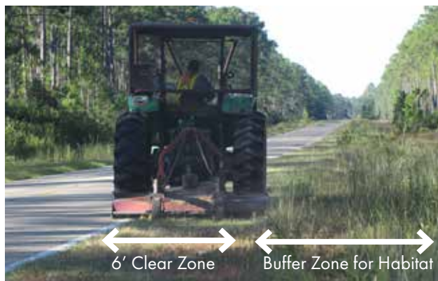
Mowing a 6-foot wide clear zone can provide roadside habitat without compromising driver safety. Photo courtesy of Jeff Norcini, OecoHort LLC.
